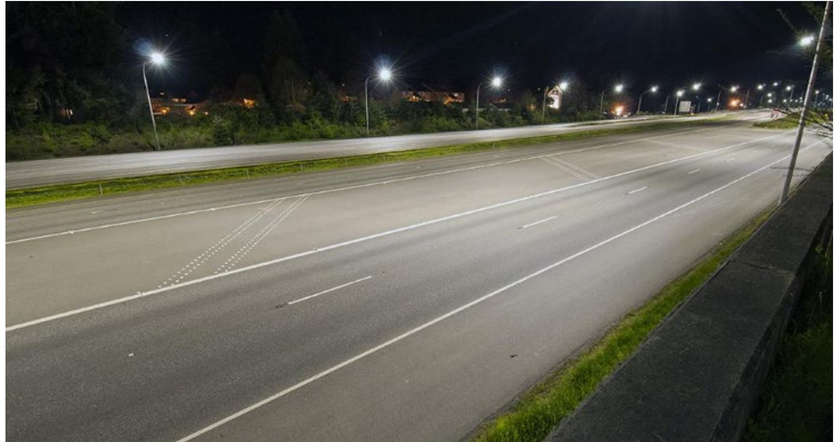
Uniform illumination with LED lighting
