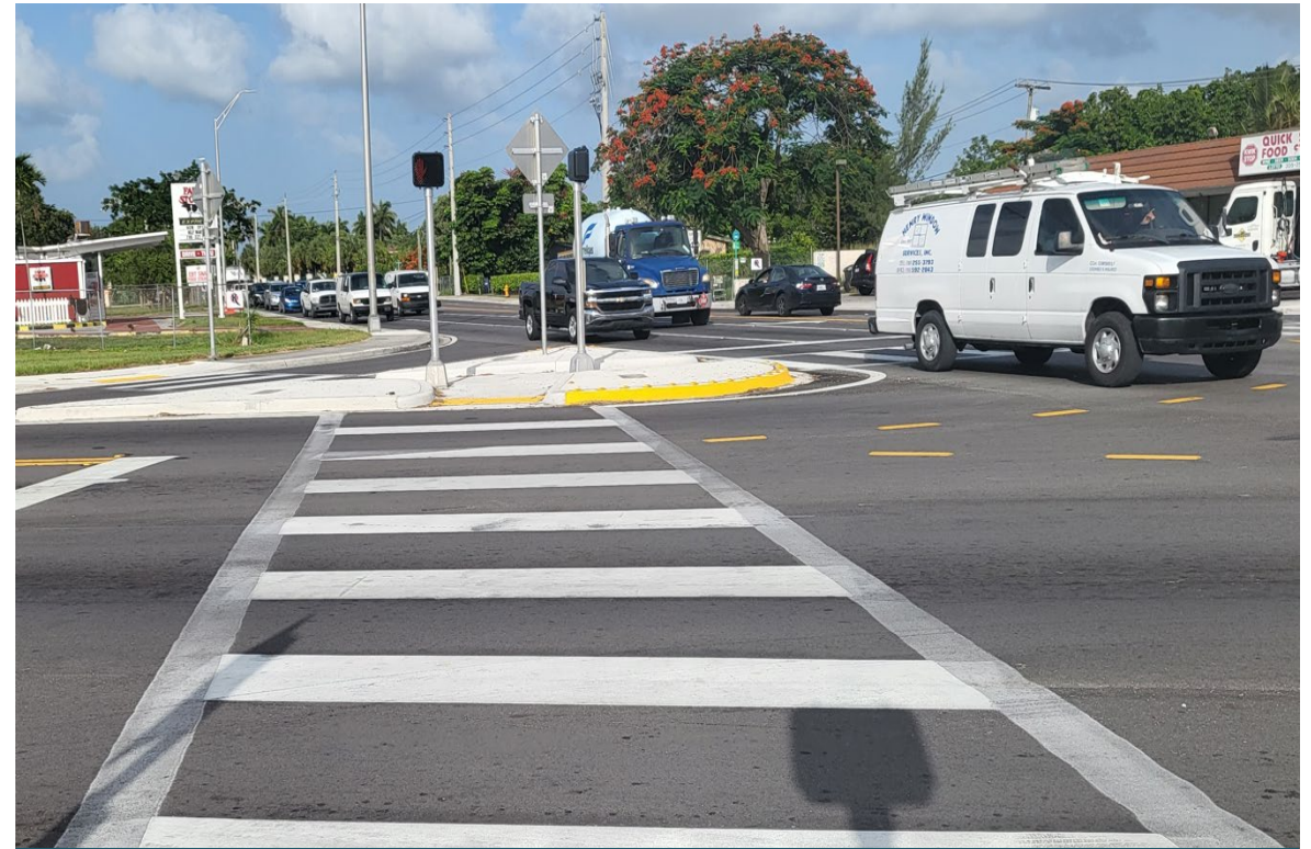
Road Recently Restriped with adequate crossing markings
