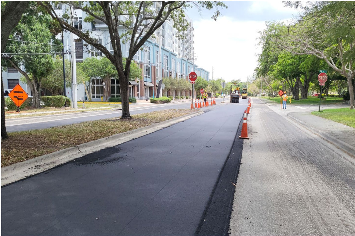
Typical Resurfacing Operation
